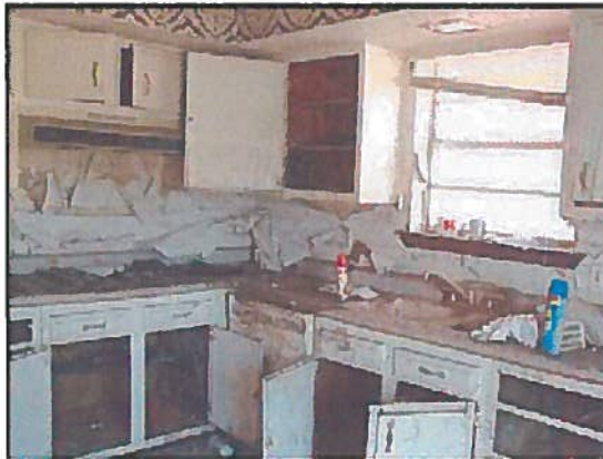
Surveying the Kitchen
